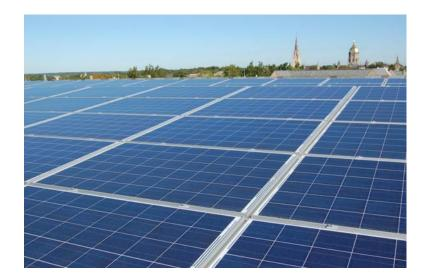
Harvesting Solar Energy at Notre Dame. 50 kW photovoltaic panels installed on the roof of Stinson Remick Hall went on operation in 2010. This new building is also the home of Sustainable Energy Institute and ND Nano
